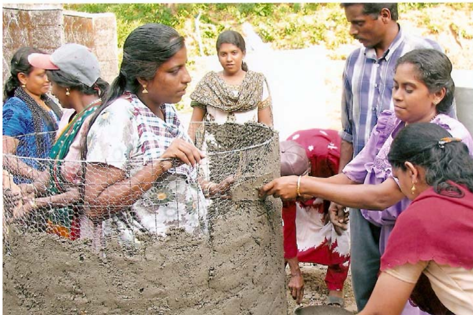
Training of women for construction of mobile biogas plant under the project "Propagation of technologies on water conservation and waste disposed through women group".
