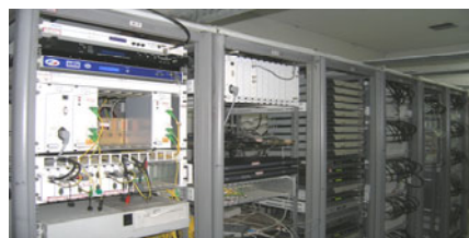
EDFA module in the main studio of Cable Comm, Saltlake, Kolkata
