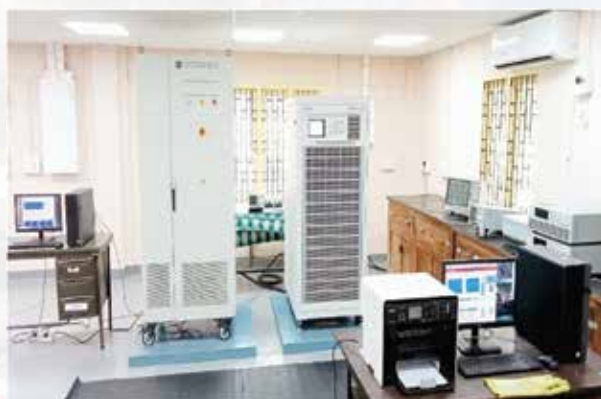
Fig. 12 Testing service facility for 30 kVA solar inverter manufacturers
