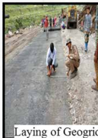
Fig.: Test Section with Geogrid placed on Subgrade (Tenga Valley, Arunachal Pradesh)
