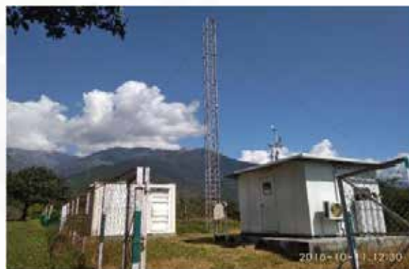
Fig. (9) CSIR-NPL's Remote Monitoring Station
