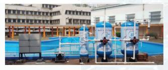
High flow rate Fluoride & Iron removal filter
