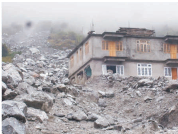
Fig. Damage due to Mudslide at Lachung
