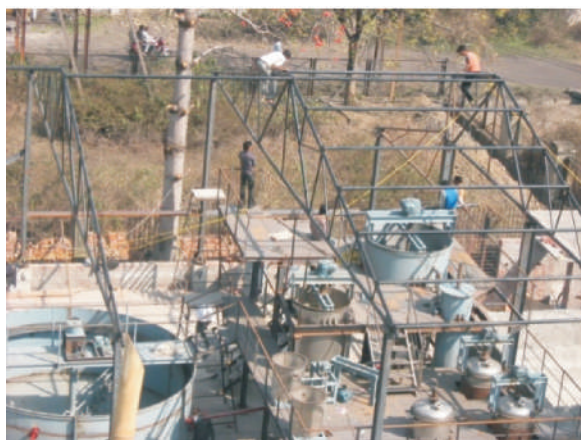
Fig. Installation of 25000 litres/day coal mine water reclamation plant in progress
