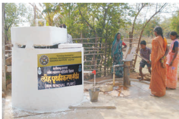
Fig. HP attachable iron removal plants installed in Durg district
