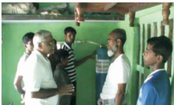
Fig. Resin-based community scale arsenic removal units installed in mosques in W.B
