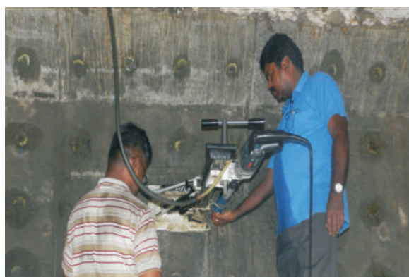
Fig. Assessment of residual prestressing force using Trepanning technique
