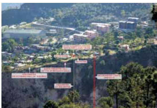
View of instrumented landslide site from Rampur side hill
