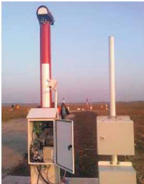
Drishti at Main Runway 28-10 of IGI Airport
